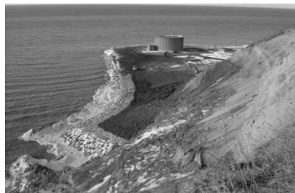
Completed Revetment
